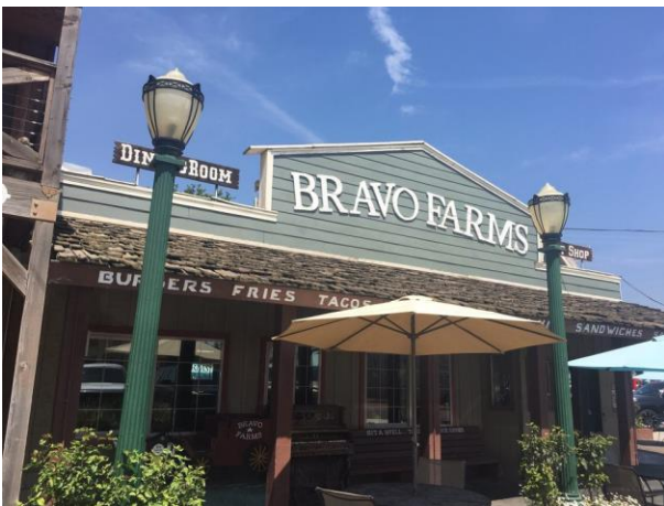
Bravo Farms – newly renovated
